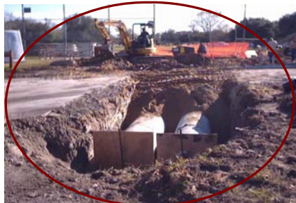
Southside System A Rehabilitation
