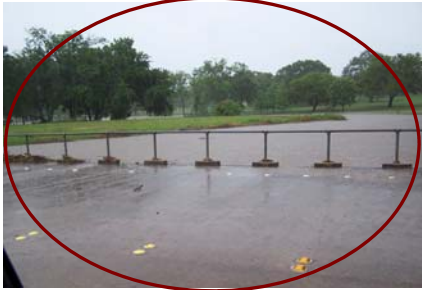
Briar Creek Flood Study
