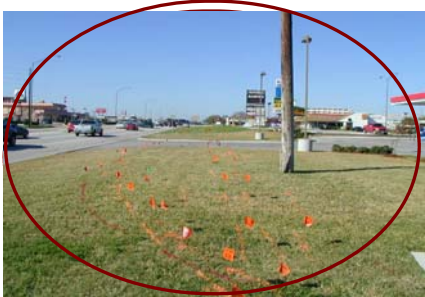
Texas Avenue Water/Sewer Relocation
