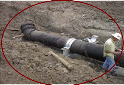
Texas A&M University Water Relocation
