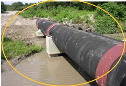
University Ranch Trunk Sewer Line
